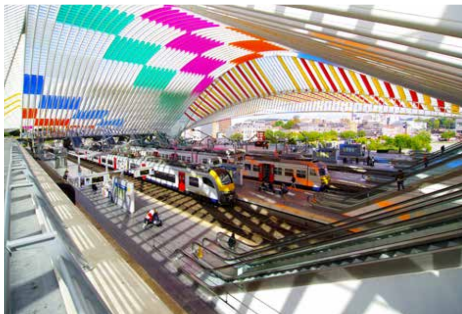
Liège-Guillemins station has one of the most spectacular roofs in Europe.
